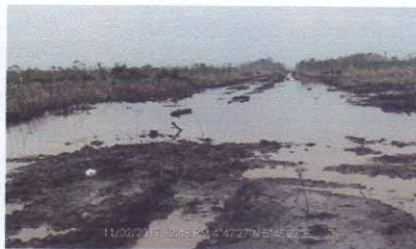
Point backfilled after repair.
